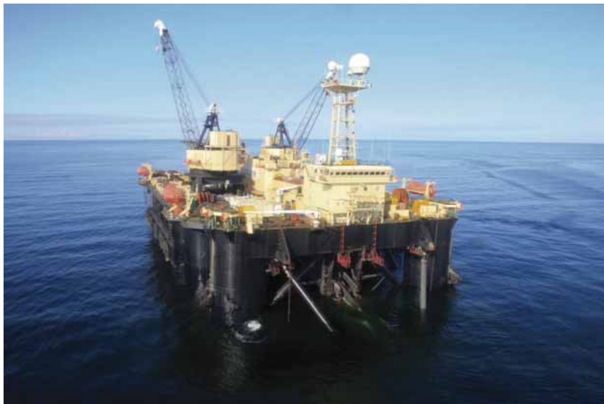
Figure 4-12. An anchored lay vessel – Castoro Sei. Photo by Nord Stream AG.
