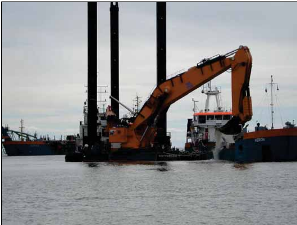
Figure 6-16 Backhoe dredger with splitter hopper barge moored alongside (right).
