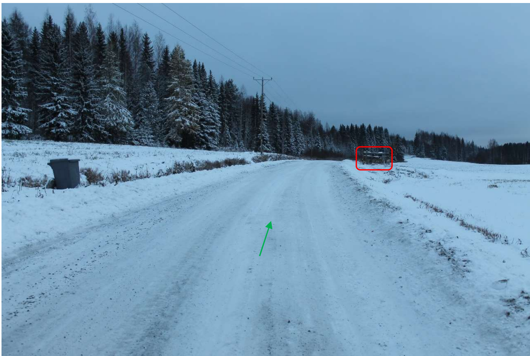
Pos 39/Pic 74. Road 16235 (Keskimmäisentie). Road need to be levelled. Road need to be fixed according to specifications for site roads. Marked mail box need to be removed. Green arrow points driving direction for Entrance B.
