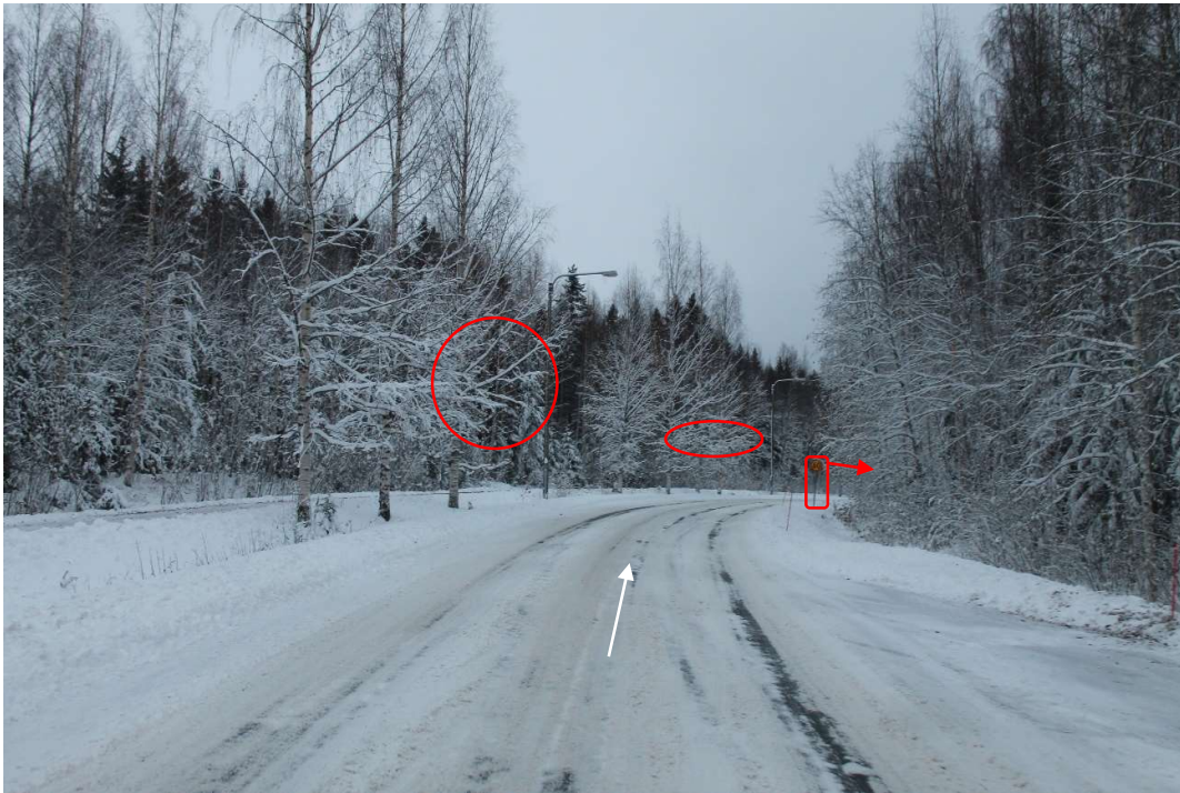
Pos 26/Pic 45. Road 16222 (Tervakankaantie). https://maps.app.goo.gl/gRJB RJcQuPe153AN8 Marked tree branches need to cut. Marked sign need to be removed.
