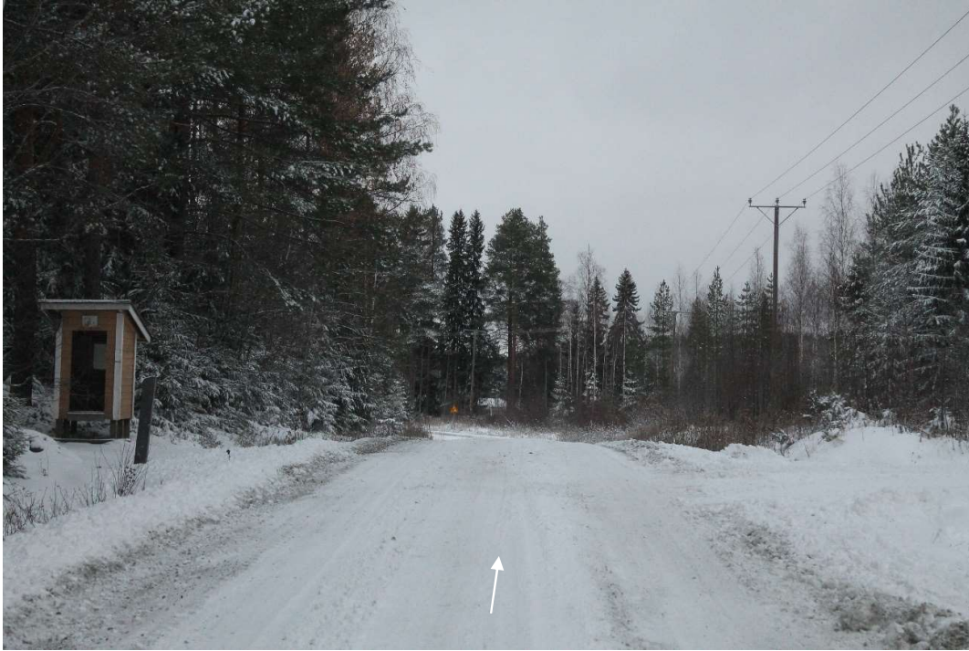
Pos 35/Pic 67. Road 16235 (Keskimmäisentie). Crest, road need to be levelled. Road need to be fixed according to specifications for site roads.
