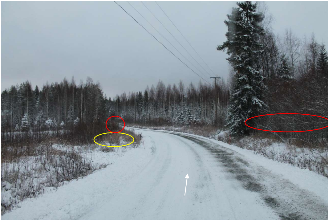
Pos 34/Pic 65. Road 16235 (Keskimmäisentie). Road need to be levelled. Marked trees need to cut. Oversail area need to be free in inner curve. Road need to be fixed according to specifications for site roads.
