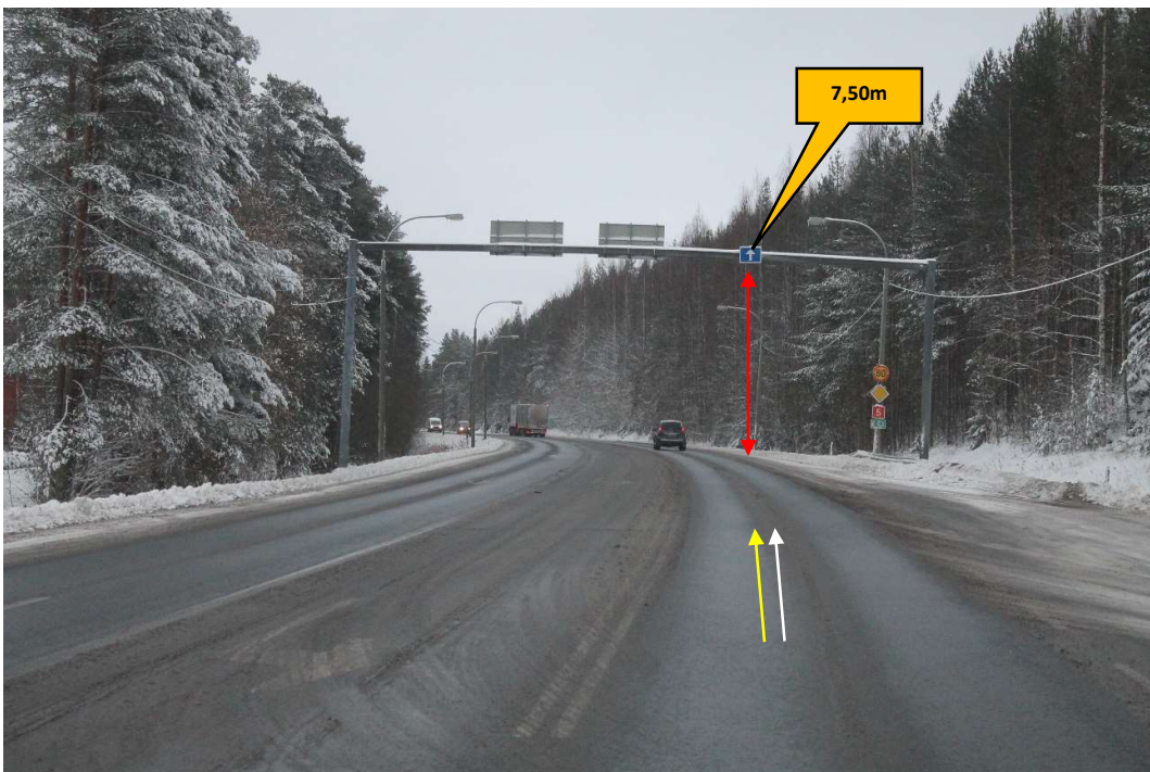
Pos 30/Pic 56. Road 5. https://maps.app.goo.gl/T6fZLTpE7Ej9am6i9 Info : Portal height 7,5m. White arrow points driving direction for route 1. Yellow arrow points driving direction for route 2.
