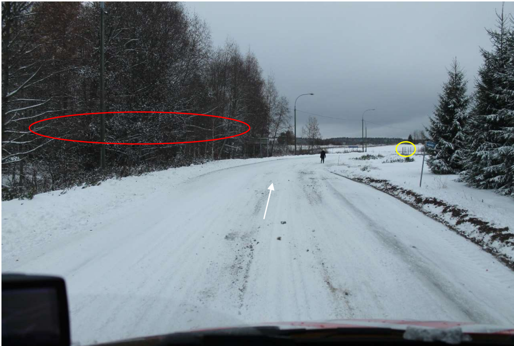
Pos 32/Pic 61. Road 16235 (Keskimmäisentie). https://maps.app.goo.gl/c3Qs88DFLQDKP1PGA Marked tree branches need to cut. Fence in inner curve close to blade.
