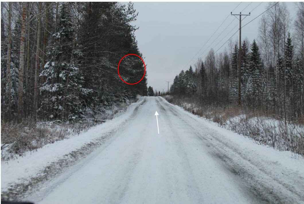
Pos 35/Pic 66. Road 16235 (Keskimmäisentie). https://maps.app.goo.gl/SRsSVNQSiambojW96 Marked tree branches need to cut. Crest, road need to be levelled. Road need to be fixed according to specifications for site roads.
