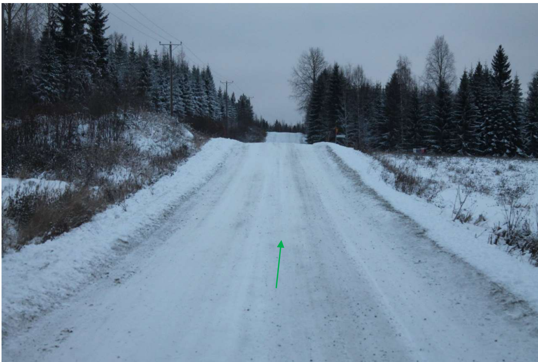
Pos 41/Pic 78. Road 16235 (Keskimmäisentie). https://maps.app.goo.gl/vq2kaHPwBVwbMojE8 Crest, road need to be levelled. Road need to be fixed according to specifications for site roads. Green arrow points driving direction for Entrance B.
