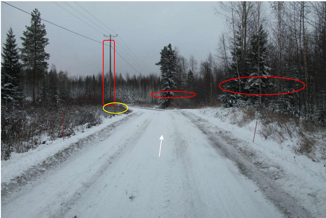
Pos 34/Pic 64. Road 16235 (Keskimmäisentie). Crest, road need to be levelled. Marked pole need to be removed. Marked trees need to cut. Oversail area need to be free in inner curve. Road need to be fixed according to specifications for site roads.
