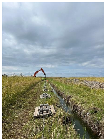
Photograph 4. Installation of the second 110kV submarine cable of the Small Strait on the coast of Muhu using the open method (Skepast&Puhkim OÜ, 21.08.2024)
