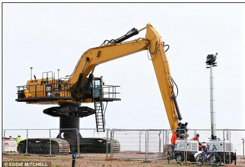
Photograph 3. Example of an excavator for the construction of a trench 3
