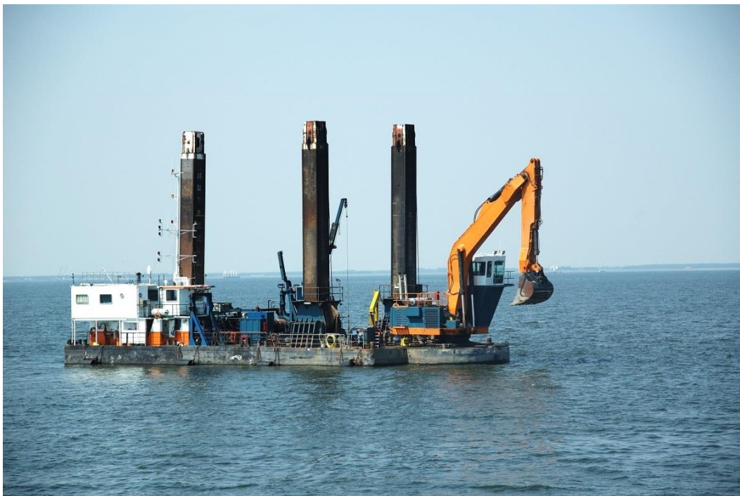
Photograph 1. Digging a trench in shallow water 2
