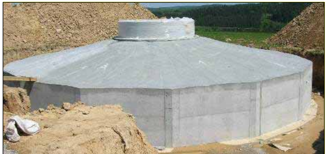
Figur 9. Gravitationsfundament.
