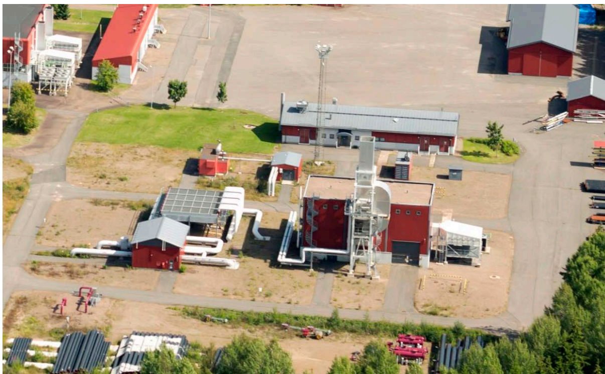
Figure 3-20. A 10 MW gas-turbine-powered pipeline compressor station in Kouvola, Finland (Gasum Corporation).
