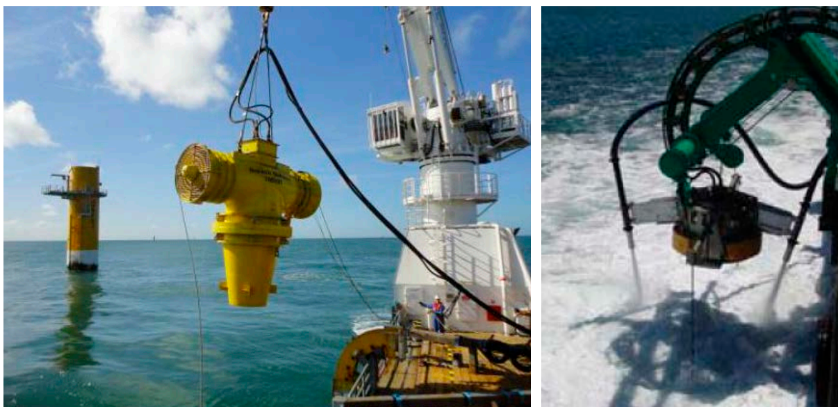
Figure 3-9. Excavation techniques using hydraulic subsea equipment: T-series digger to the left, clay cutter to the right. (Ramboll 2014a)
