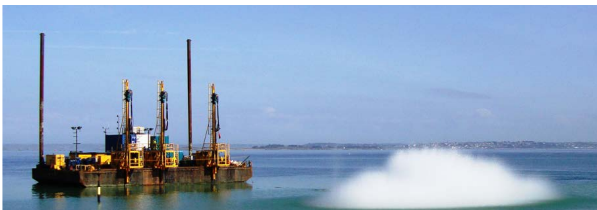
Figure 3-10. Controlled subsea rock blasting. (Ramboll 2013a)
