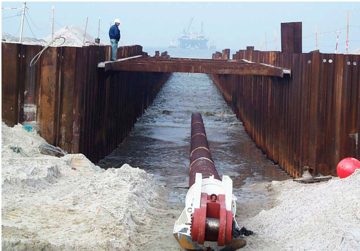
Figure 3-15. Pull head emerging from the sea at shore pull. (Ramboll 2014a)
