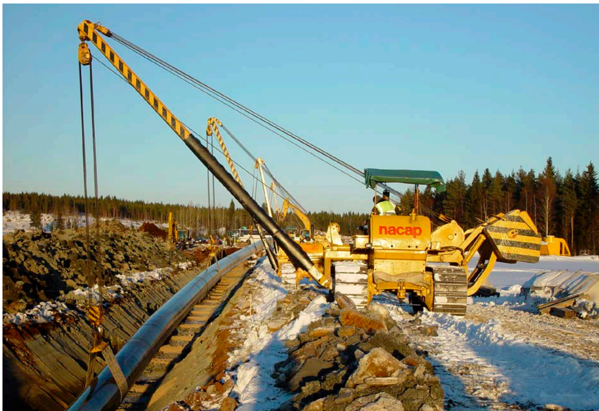
Figure 3-19. A natural gas pipeline section being laid. (Gasum Corporation)
