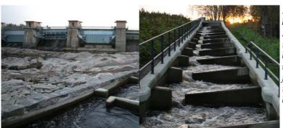
Hydromorphological pressures on rivers have major impacts on fish populations. At the city of Oulu in the Finnish pilot river basin a dam and hydropower plant built in the 1940s led to the loss of the salmon population. The construction of a fish ladder in 2000 has enabled salmon to re-established a population above the barrier.
